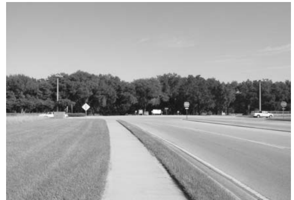
Bike Lanes will be part of the future extension of Gornto Lake Road.
