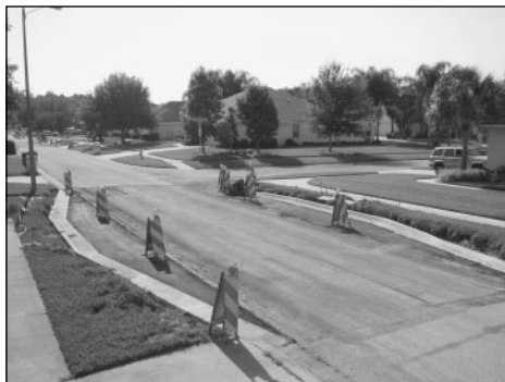
Neighborhood traffic calming devices are being installed to slow traffic on residential streets in this neighborhood in South Hillsborough County.
