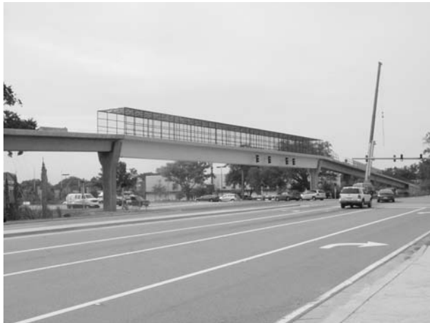
The Gunn Highway Overpass, scheduled to open in November, will provide safe crossing over Gunn Highway.
